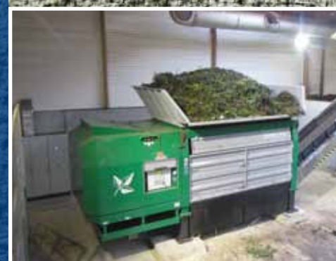
The facility in Réau treats the waste of 300,000
